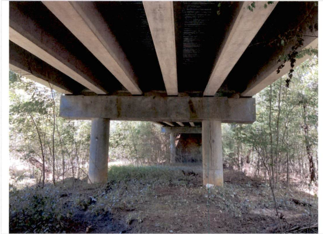
Underneath, looking at bent 2. 2024
