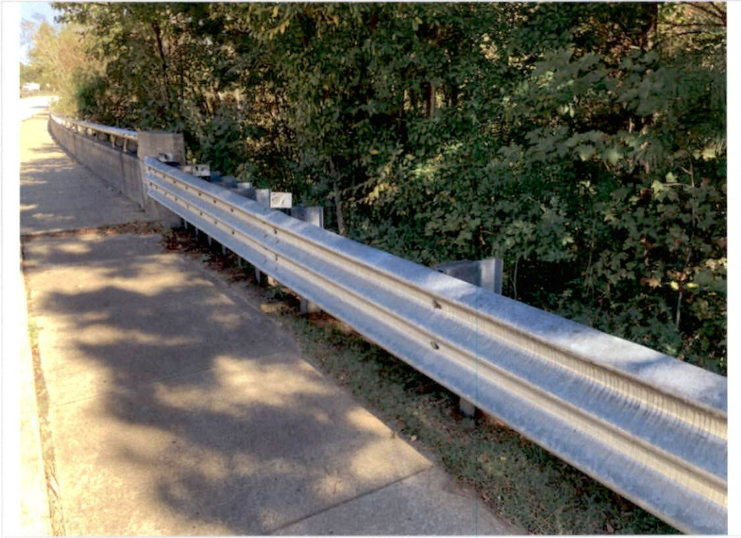
Typical guard rail transition. 2024.
