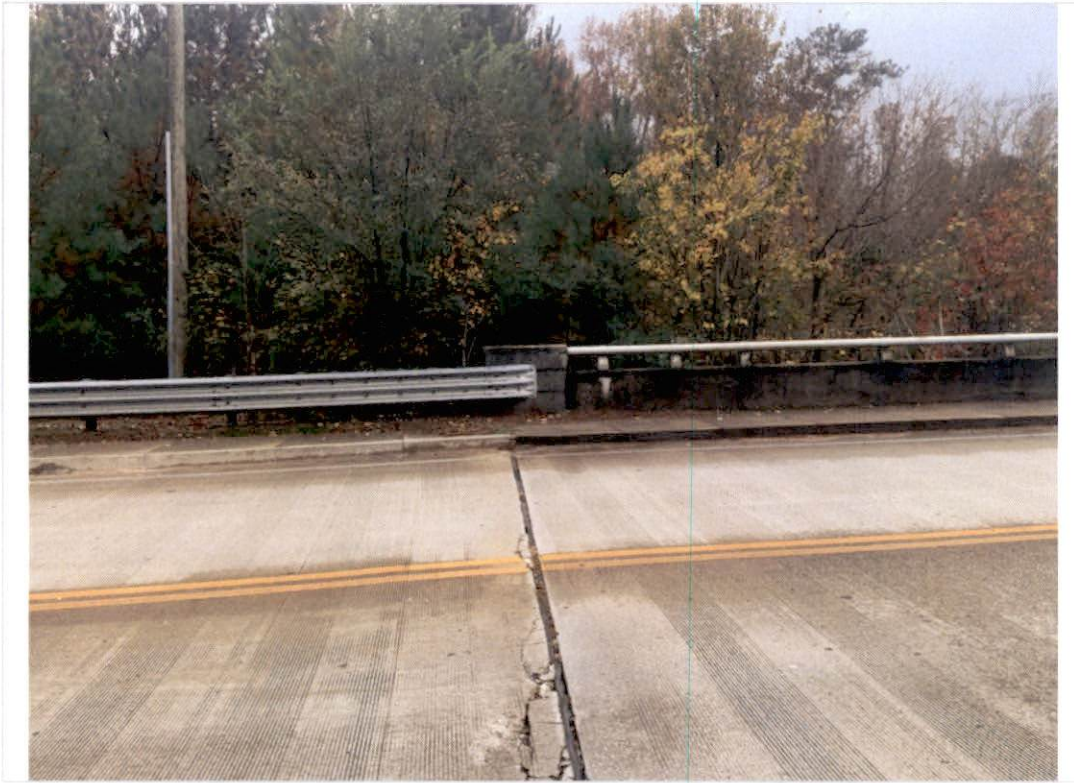
Typical bridge rail transition. 2022
