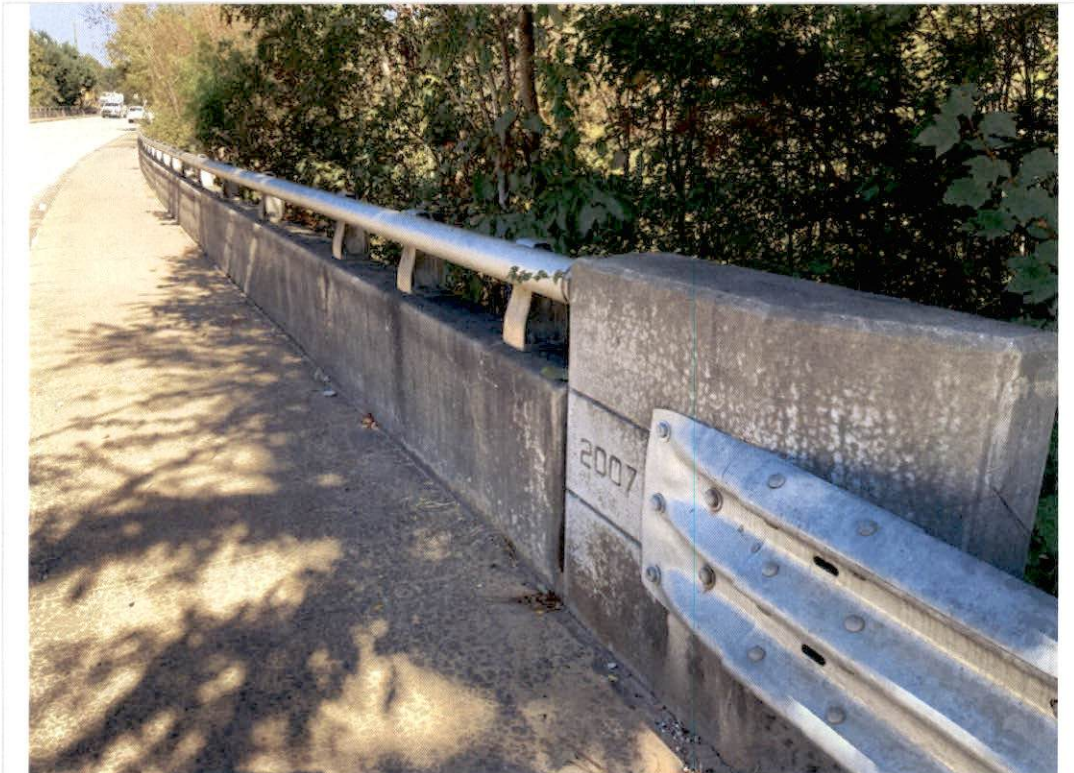
Transition connection and typical bridge rail. 2024.
