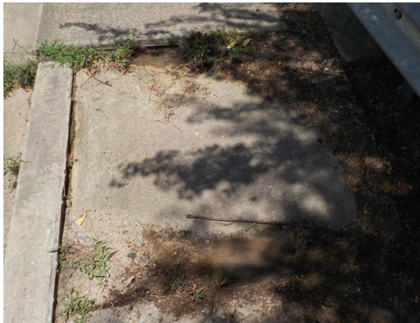
Photo 4 - 3 ½" settlement of sidewalk at southeast corner (5'-3" L x 5'-3" W x 3 ½" H)
