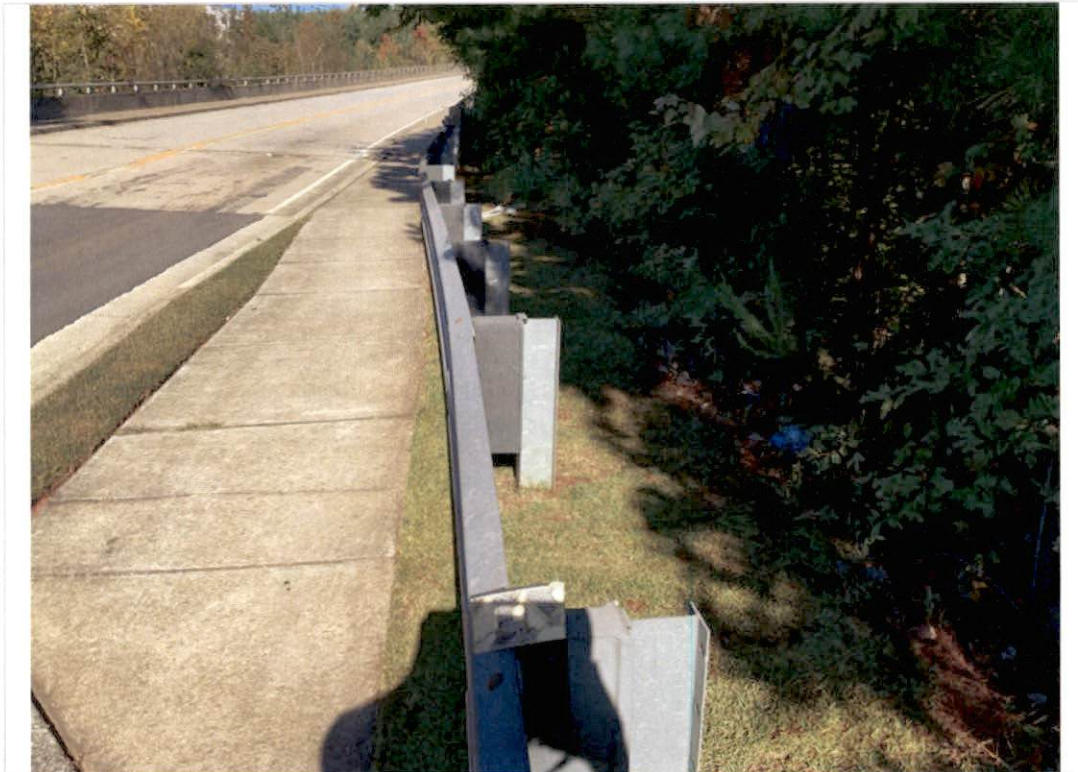
Approach guard rail. 2024
