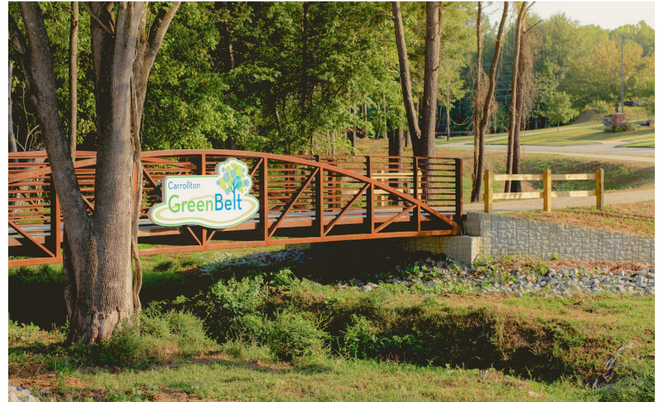
Prefabricated steel bridge trail crossing above existing roads and waterways.
