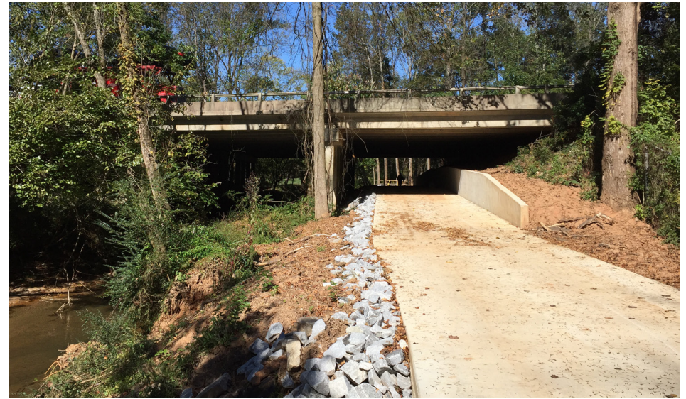
Multi-use trail going under a roadway
