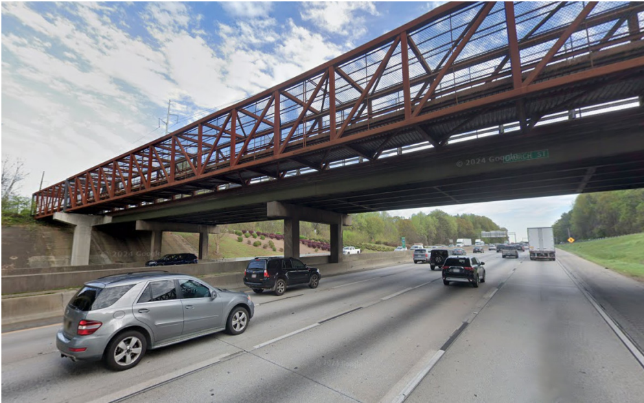
Prefabricated steel bridge allows the trail to cross above existing highways or railroads. Bridge over I-285 Stone Mountain Trail
