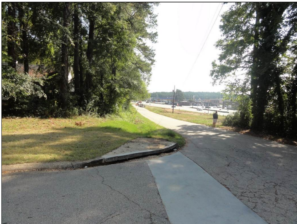
View toward the subject facing south along Gilbert Road.
