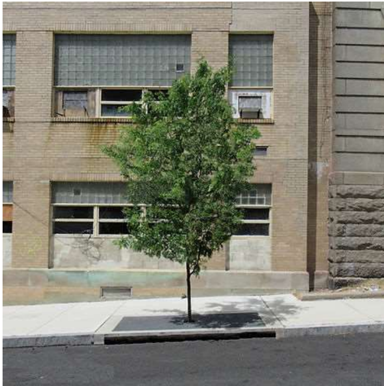
Figure 3: Example of stormwater tree well
