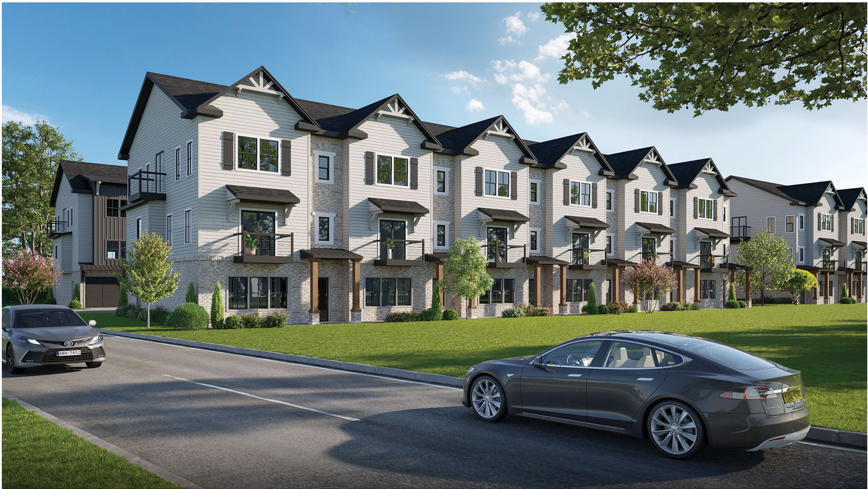
VIEW FROM EAST ATLANTA ROAD
