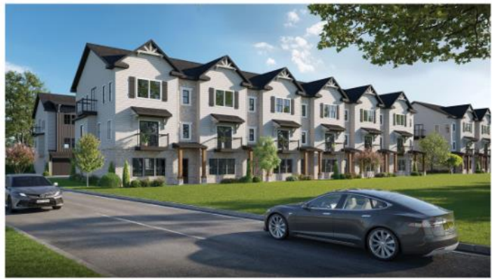
VIEW FROM EAST ATLANTA ROAD
