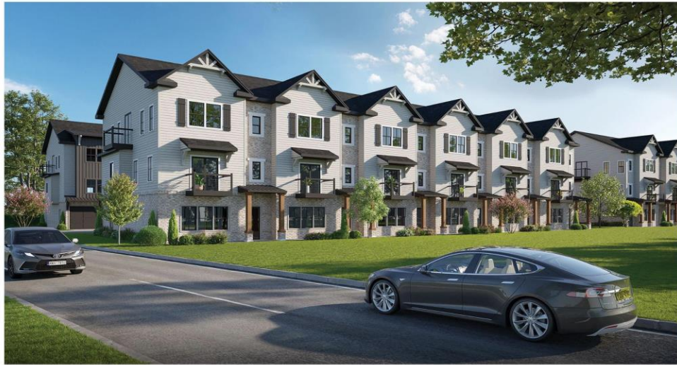
VIEW FROM EAST ATLANTA ROAD
