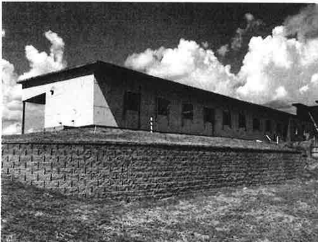
Rear elevation showing retaining wall and admin area
