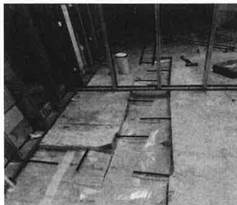
Trenches for new plumbing
