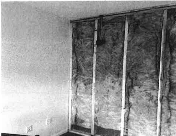
Insulation and fire alarm installed
