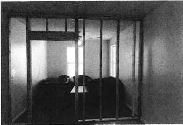
Wood framed walls installed
