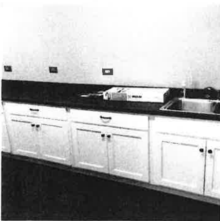
New Cabinets Installed
