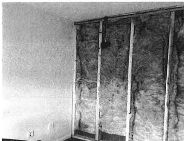
Insulation and fire alarm installed
