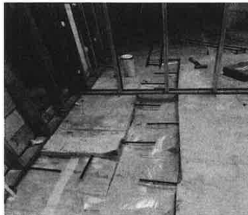
Trenches for new plumbing
