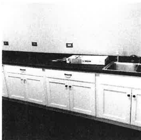
New Cabinets Installed
