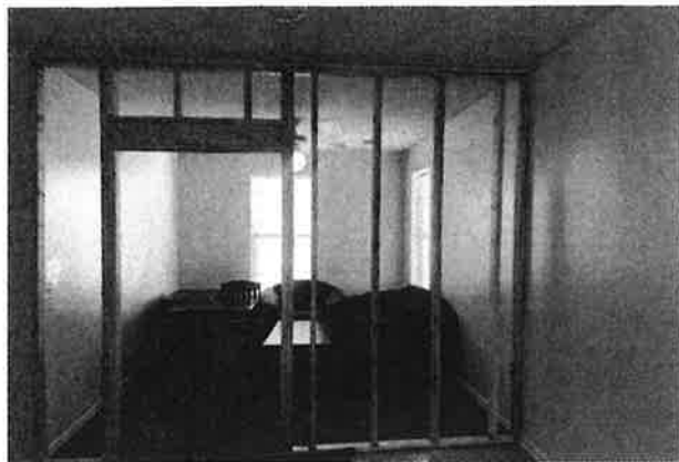
Wood framed walls installed
