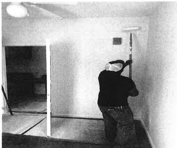
Finish Paint being applied to the new walls
