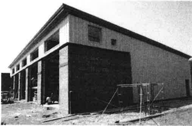
Front elevation showing PEMB apparatus bay
