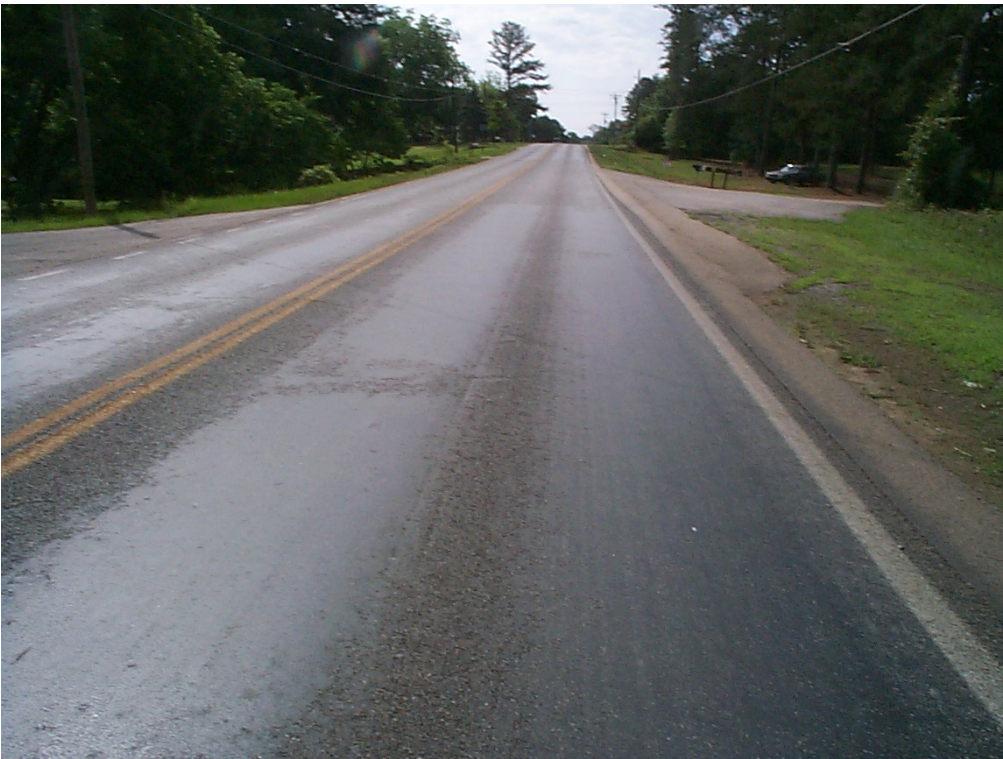
Level 2 – surface is black with very little aggregate noticeable
