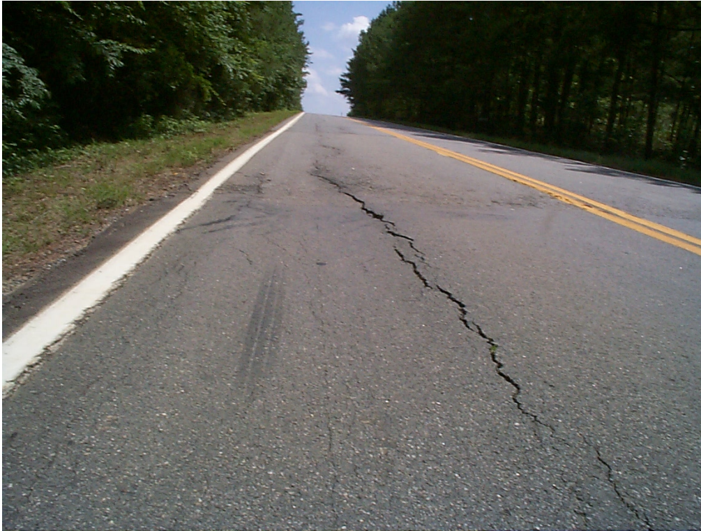
Level 2 ( Moderate) – Heavy swaying of vehicle. Fair control of vehicle, driver has to anticipate dips ahead
