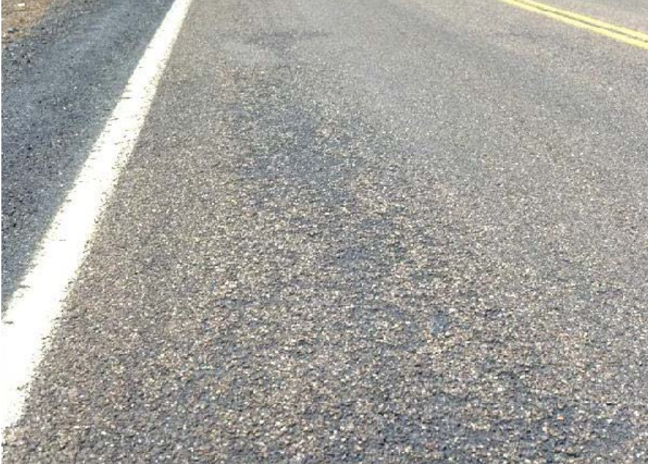
Level 2 – loss of most surface
