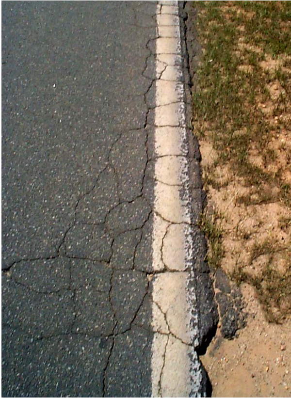
Level 2 – crack widths greater than \frac{1}{4} inch, double cracking, tight “alligator” cracking
