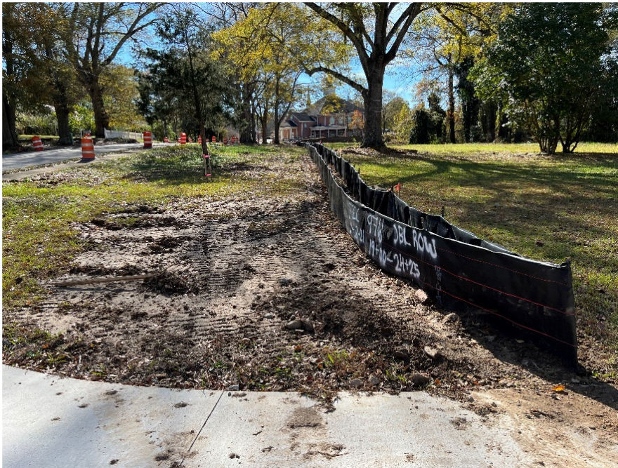
Silt Fence Installation
