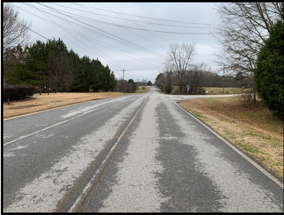
Photograph 3 – Brannan Road Facing North at North Salem Road
