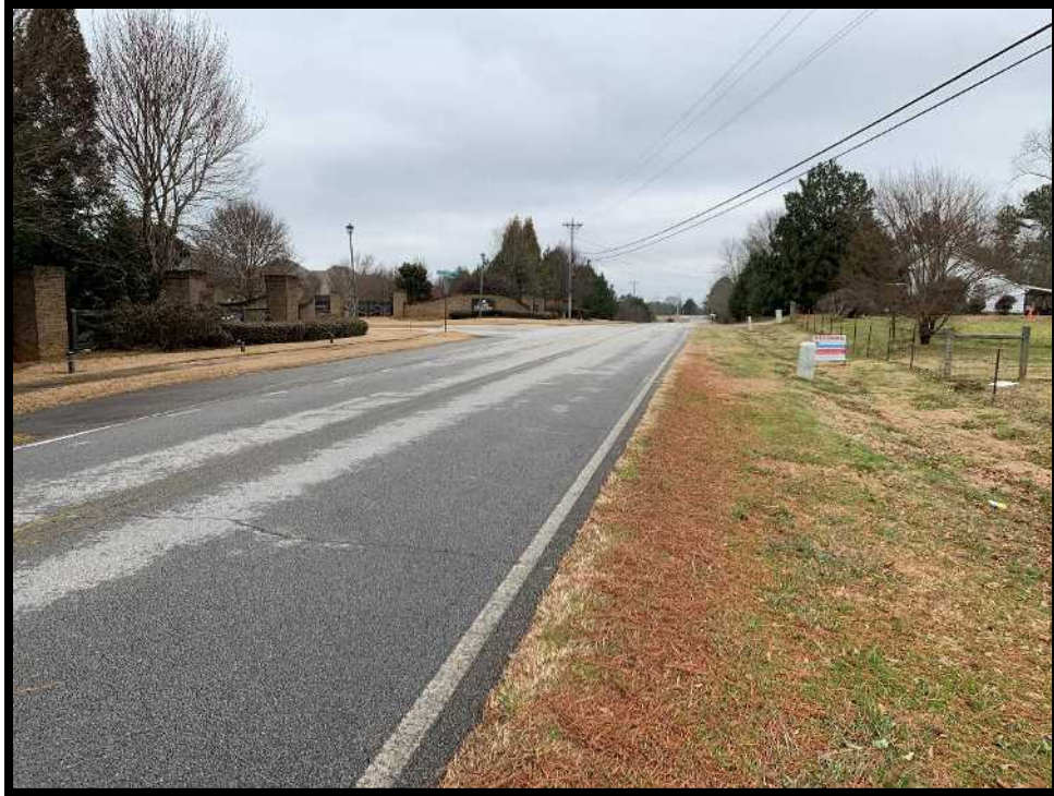
Photograph 1 – Brannan Road Facing North at Sprayberry Lane (Site to Right)
