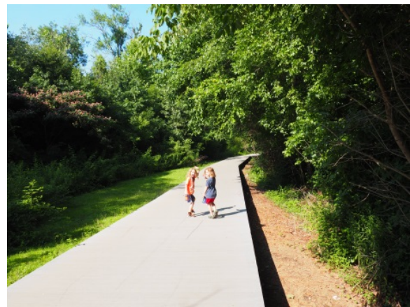
Figure 16: Elevated boardwalk multi-use trail.
