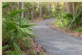
Off-road soft surface multi-use trail
