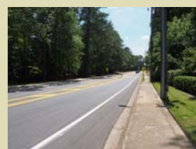
Sidewalk with no buffer
