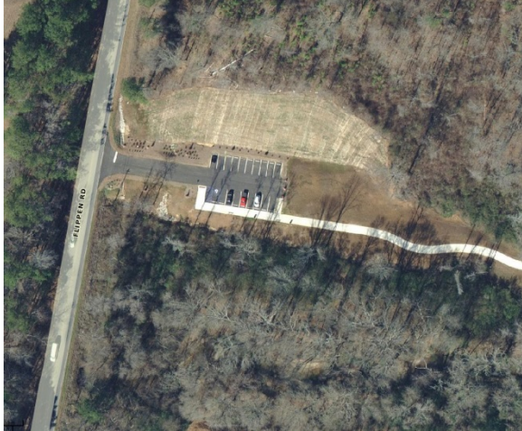
Figure 12: Parking for Reeves Creek Trail off of Flippen Road. The trail route follows a creek, sewage, and power easements.
