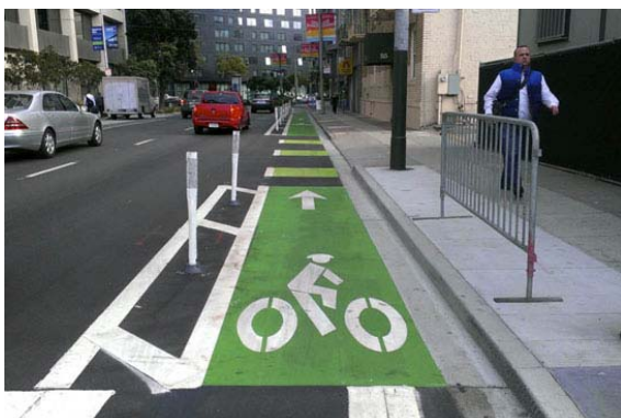
Figure 21: Separated bike lane. ( https://www.fhwa.dot.gov )
