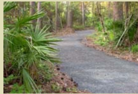
Off-road soft surface multi-use trail
