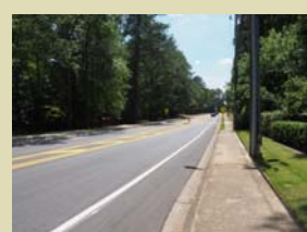
Sidewalk with no buffer
