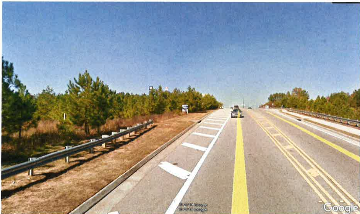
Site view looking to the North
