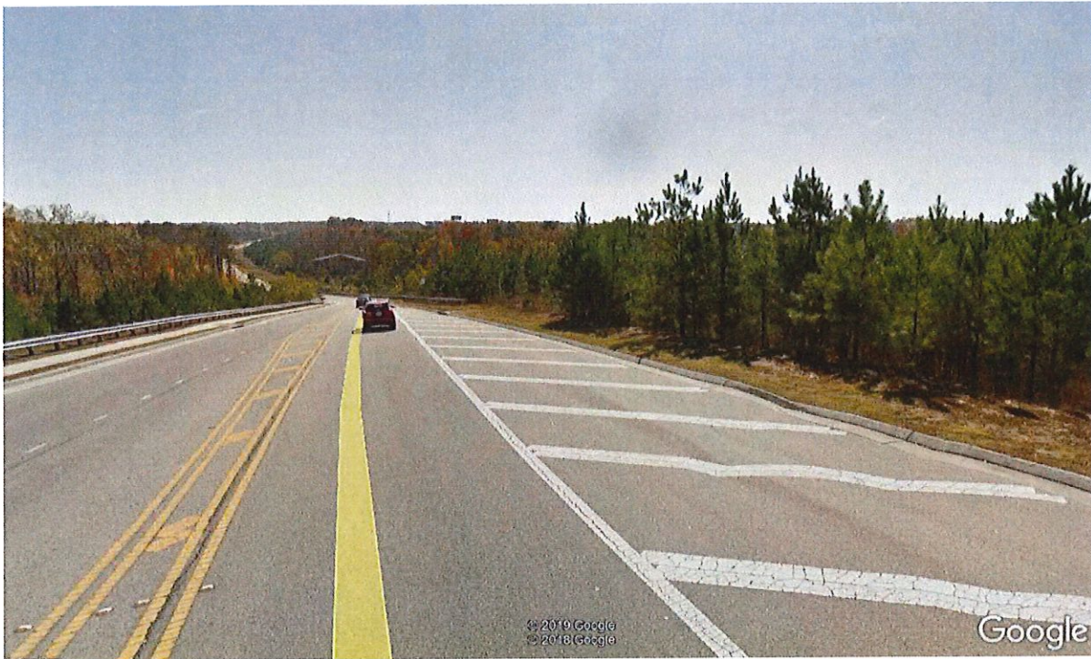
Site view looking to the south
