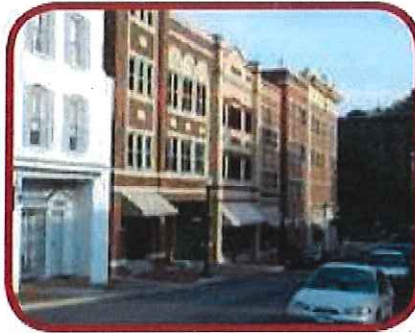
Entrance integrated into architecture of the facade
