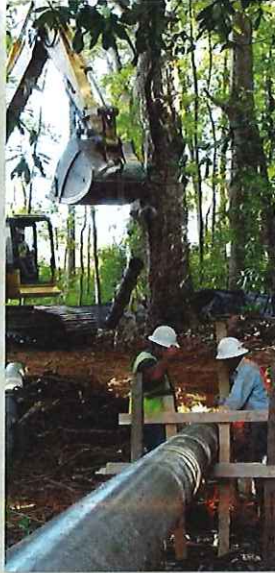
Water/Wastewater & Stormwater Management
