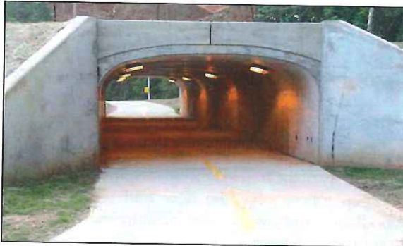
Bike and Pedestrian Tunnel under Webb Bridge Road
