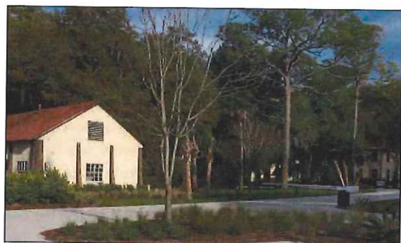
Consolidated parking area in Historic District
