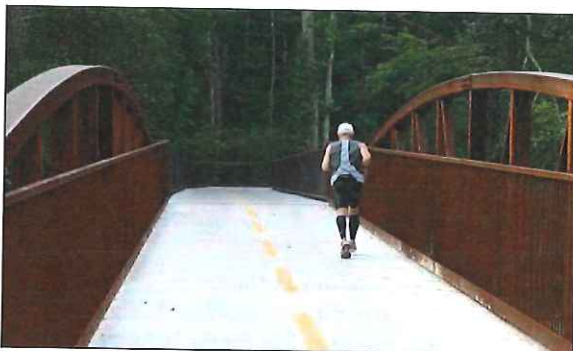
Bike and Pedestrian Bridge over Big Creek
