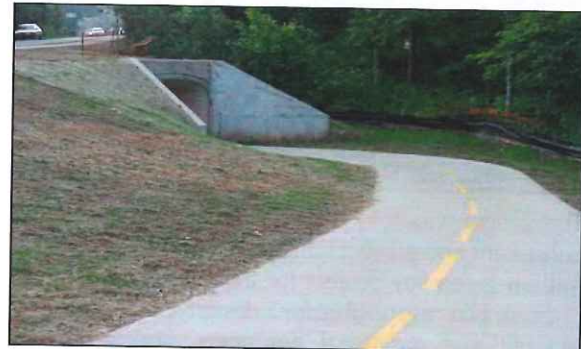
Trail Approach to Tunnel with Webb Bridge Road Above
